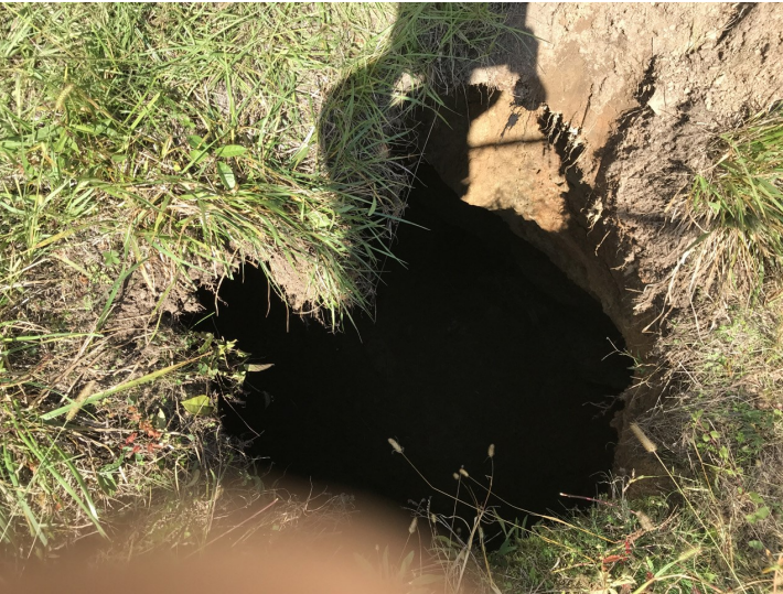
The Walker Circle Subsidence Emergency project developed from a discovery by a right-of-way grass cutting crew in the City of Dora. A site evaluation revealed an approximate three-foot diameter hole extending down to a depth of approximately eight to ten feet below grade where it encounters the apparent remnants of old mine works. The road was closed and traffic rerouted until the subsidence could be repaired.
