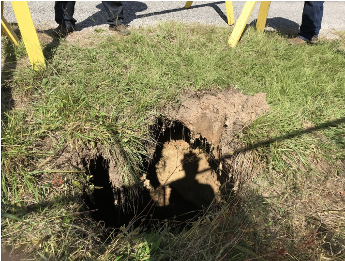
The Walker Circle Subsidence Emergency project developed from a discovery by a right-of-way grass cutting crew in the City of Dora. A site evaluation revealed an approximate three-foot diameter hole extending down to a depth of approximately eight to ten feet below grade where it encounters the apparent remnants of old mine works. The road was closed and traffic rerouted until the subsidence could be repaired.
